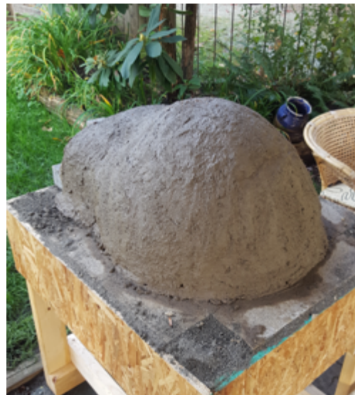
Inner layer of the cob oven, formed over sand
